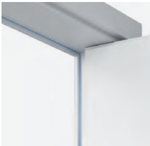
Door frame corner from hinges side
