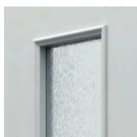
glazing bead with a glass panel
